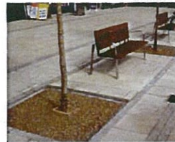
Stabilised decomposed granite to tree pits; revised from corten steel grates
