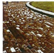
Feature pavement: used brick sourced from site; revised from proposed art components in paving
